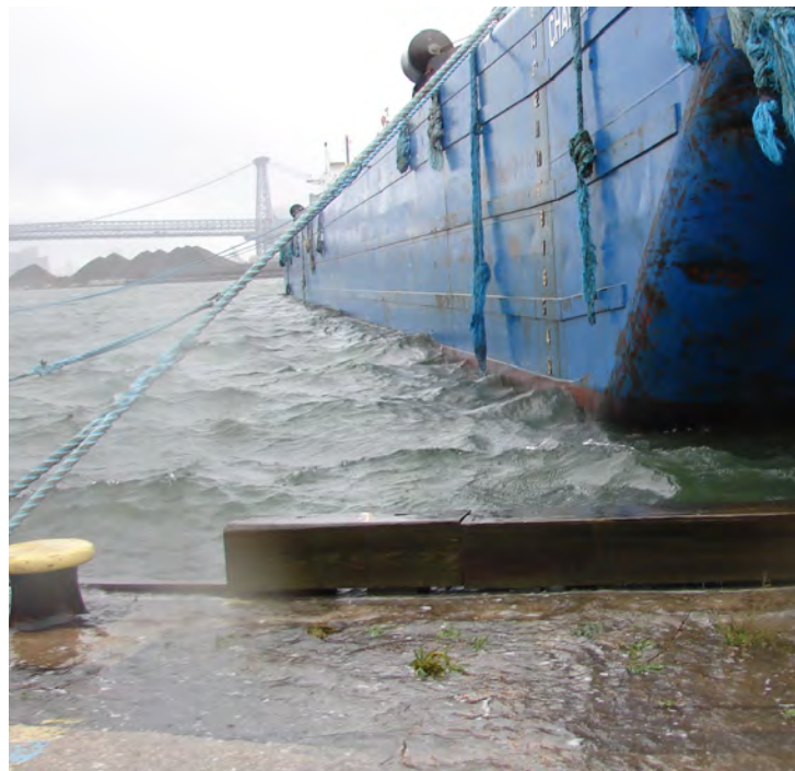
Flooding at the berths during Superstorm Sandy
