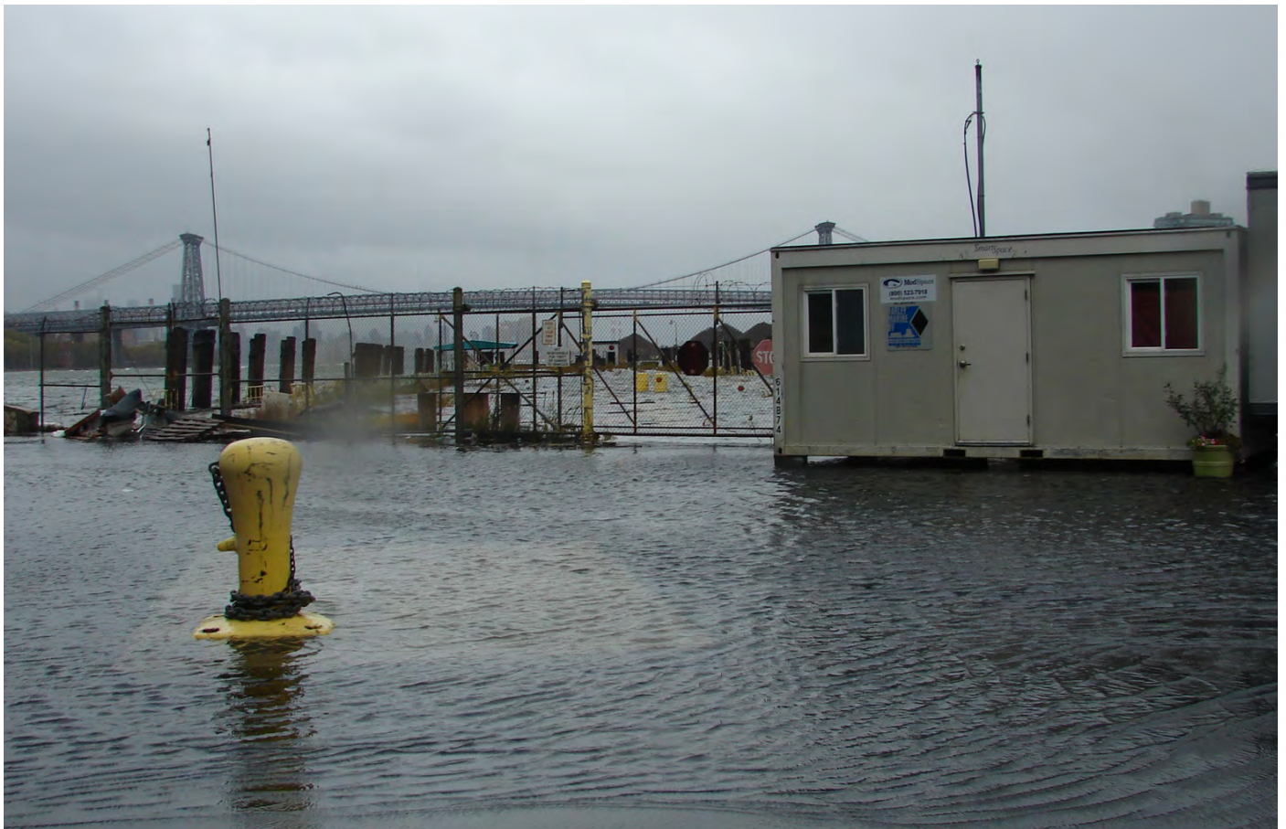
During Superstorm Sandy in October 2012, areas of the Yard were inundated with four to six feet of water, which penetrated substations, basements, ground floors and lobbies, boilers and boilers housings, and dry docks.
