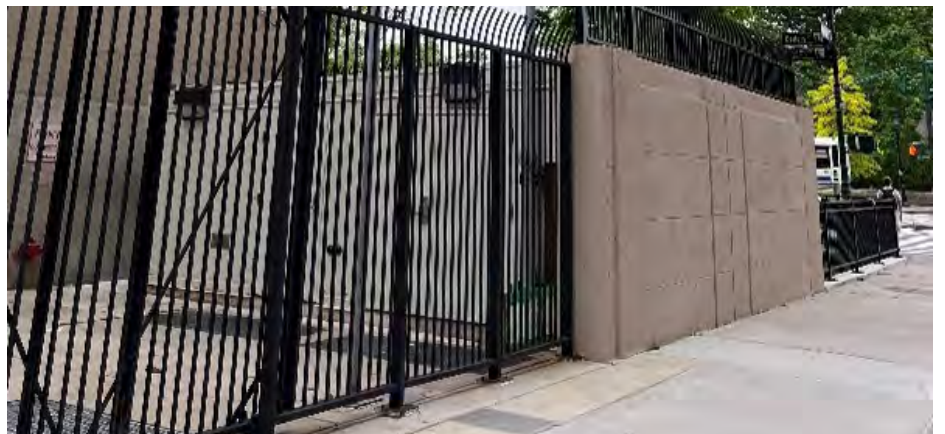
Sliding or Deployable Gates
