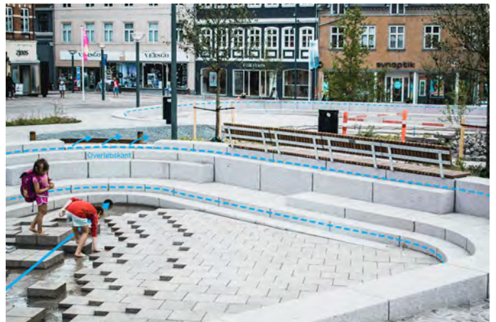
Figure 30. Blue-Green Infrastructure (BGI) Hardscape Plaza in Ringsted Torv, Denmark
