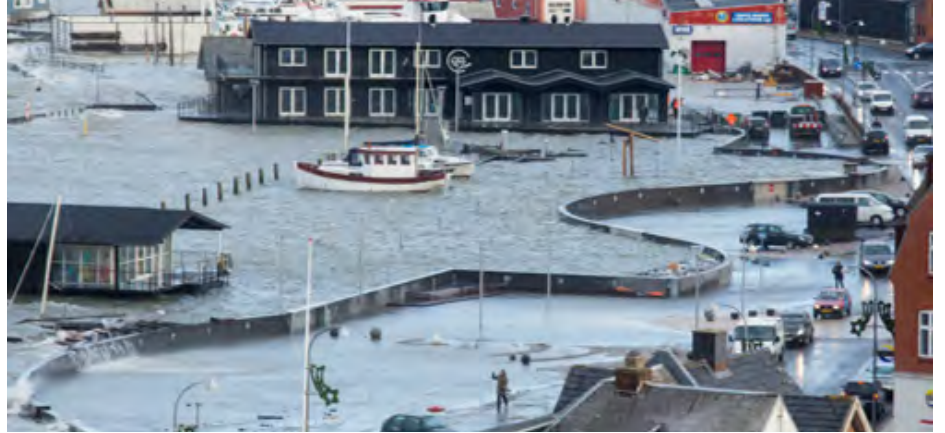
Concrete Flood Walls
