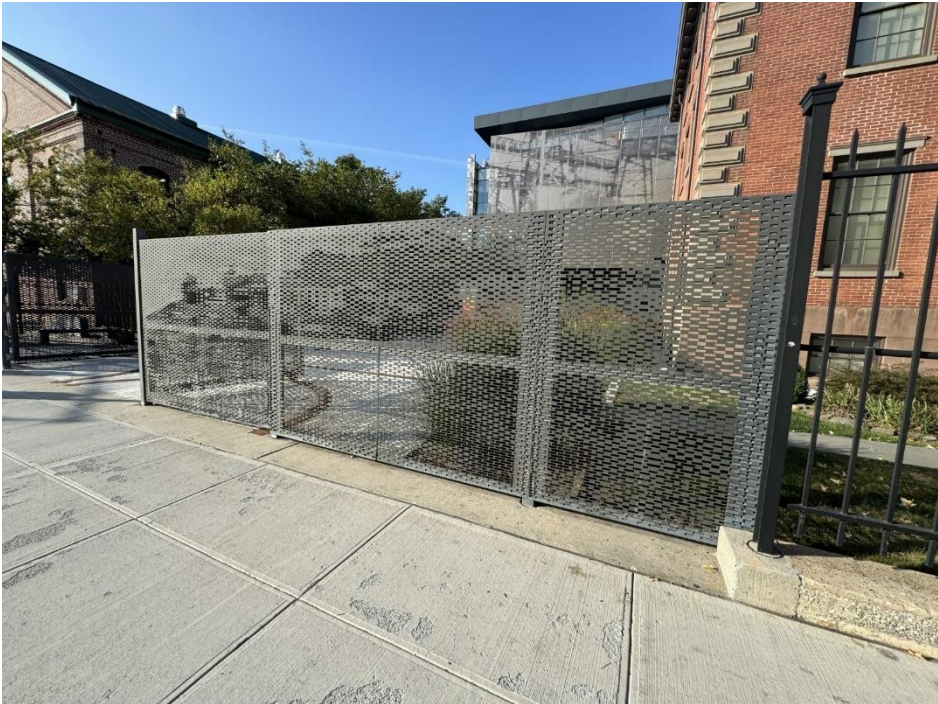
Three panels of CNC designed fence: 26' W x 75" H. Sections C49-51
