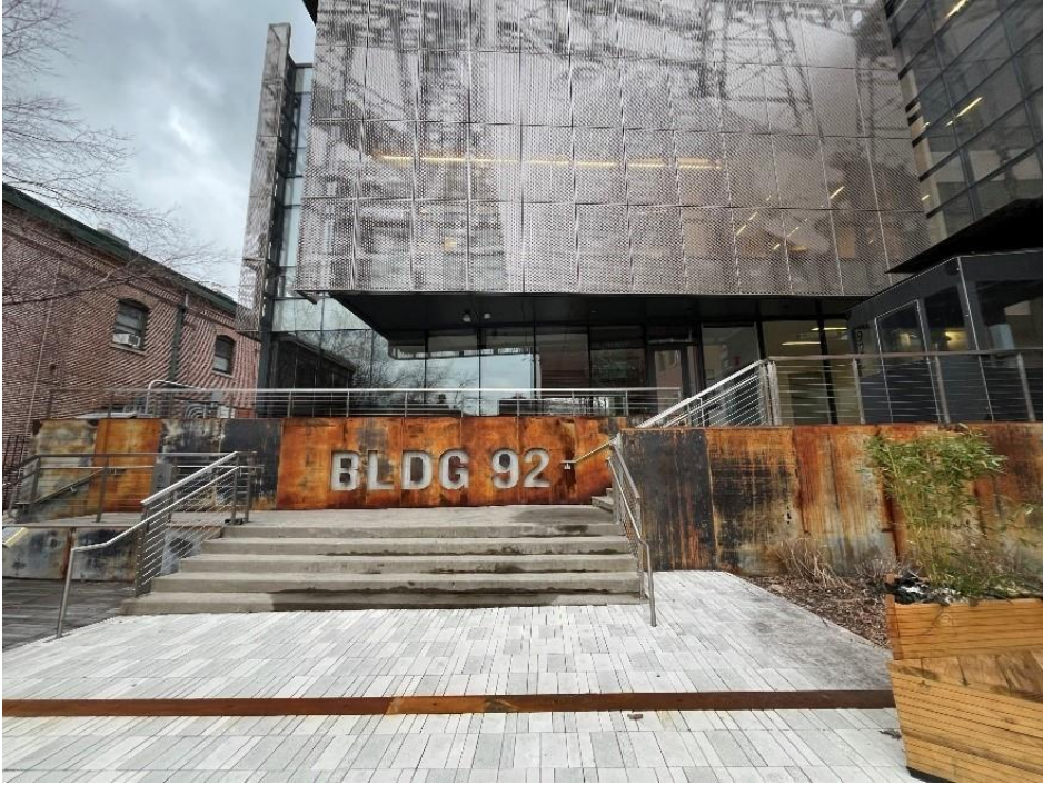
Front façade of Building 92
