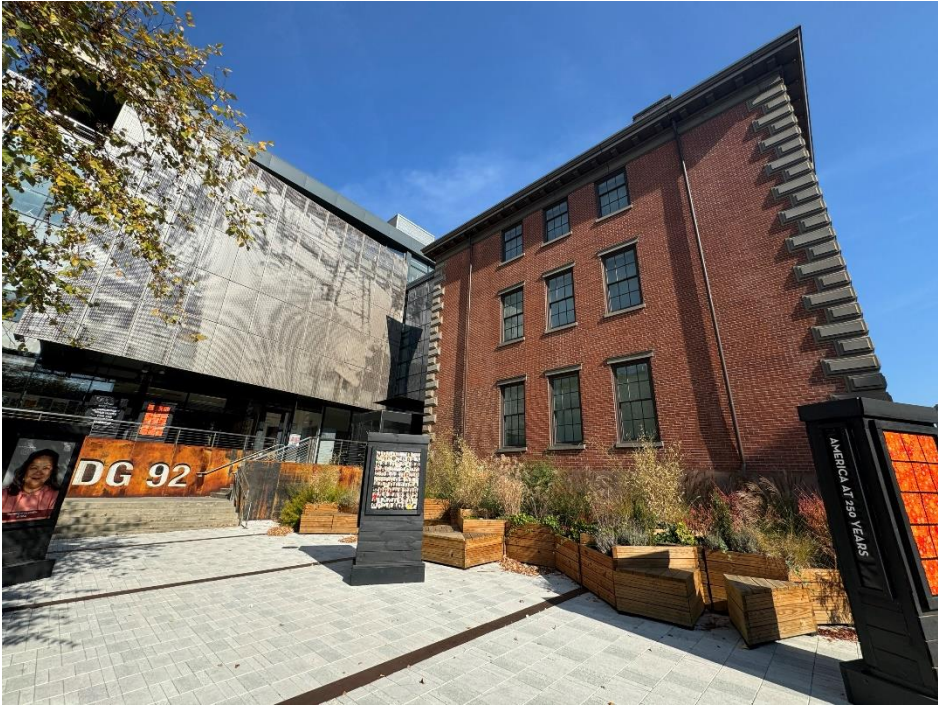
Right-side courtyard in Building 92 forecourt; Courtyard: 70' L x 62' W
