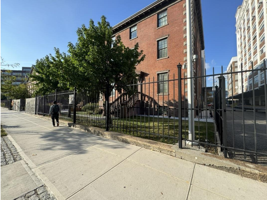
Five panels in front of Historic Marine Commandant's House at Building 92: 54' W x 82" H. Sections C44-48
