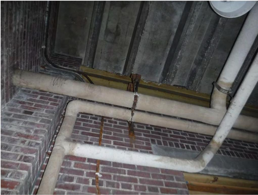
386B – ACM Pipe Insulation Jacket Mud fill, Pipe Insulation Jacket Lagging & Pipe Insulation Elbow to Fiberglass
