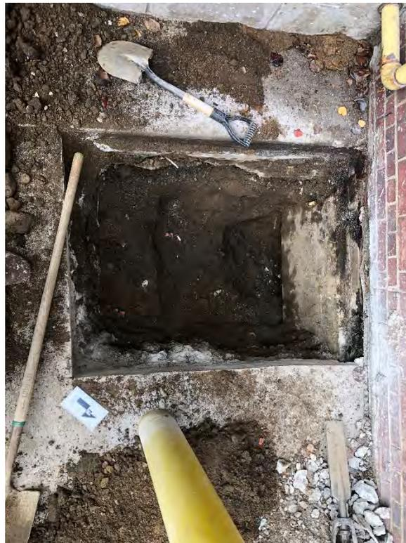
**Photo 10:** Test Pit TP-62-1 upon encountering bottom of footing (facing southwest)
