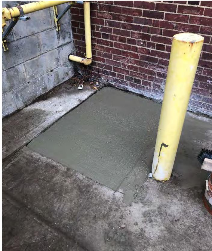
**Photo 11:** Test Pit TP-62-1 after backfilling and concrete patch (facing west)
