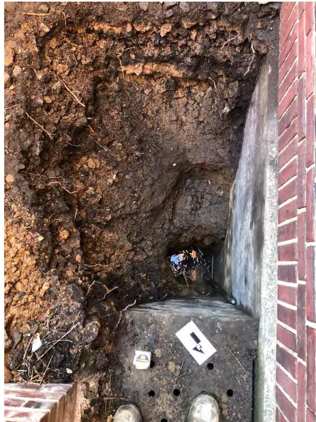
**Photo 18:** Test Pit TP-386-1 upon completion (facing southwest)
