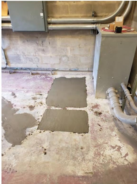
**Photo 16:** Test Pit TP-293-1 after backfill and concrete patch (facing northwest)
