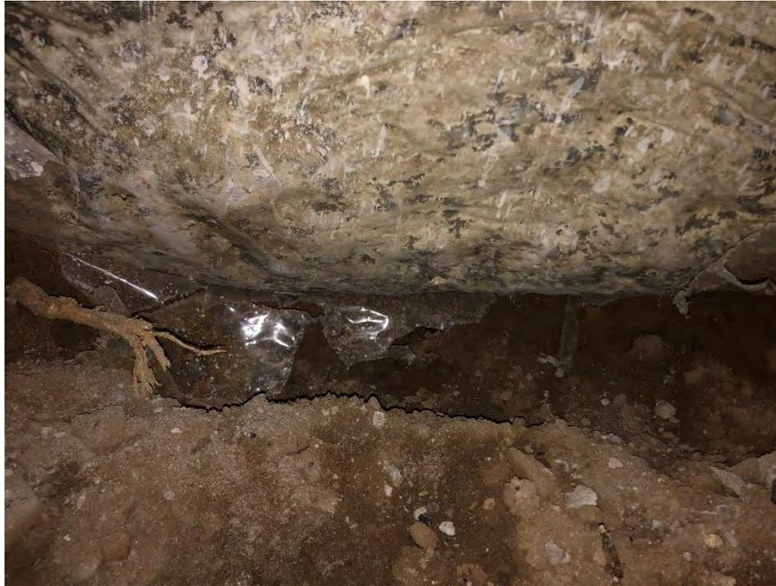
**Photo 15:** Test Pit TP-293-1 waterproofing along northwest wall (facing northwest)
