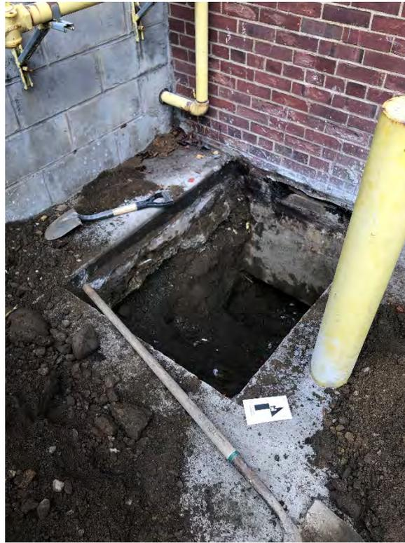
**Photo 9:** Test Pit TP-62-1 upon encountering bottom of footing (facing west)
