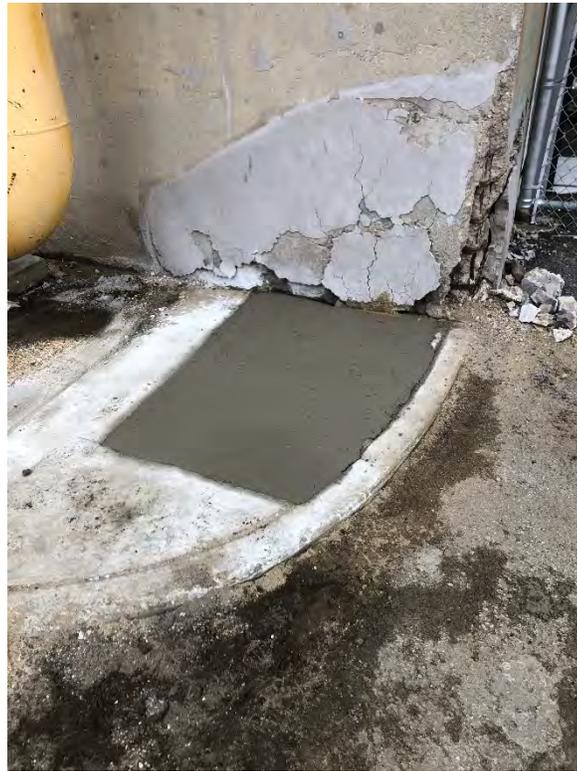
**Photo 3:** Test Pit TP-41A-1 after backfilling and concrete patch (facing east)
